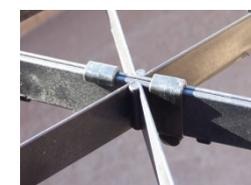
Grids should be placed so that the diagonal lines in the grid match up across the whole of the grids - i.e. consistent throughout the grid work. Grids can be staggered to minimise waste. As long as the diagonal lines are maintained, the grid can be positioned anywhere on the beam.
