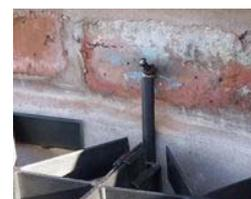
If you are securing the support line with ceiling anchors, you will need to drill a suitable hole with a 6.0mm masonry drill bit. Then gently tap the ceiling anchor into the hole, leaving only the hole in the ceiling anchor exposed. To ensure that this hole remains open, you can temporarily place a spare ceiling anchor into this hole whilst tapping the fixing into place.
