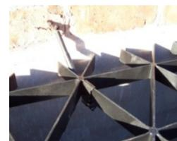
Check again that the area of pond base is level at the point where the foot rests. The SafaDeck will be more secure if a single grid crosses any joints in the beam. It is recommended that all legs supplied are used.
