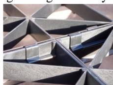
Grids are clipped to the beam using beam clips. The beam clips are placed in each corner of the grid. Beam clips are placed tab down. The top of the clip needs to be placed on top of the grid and then the clip pushed into place onto the beam.
